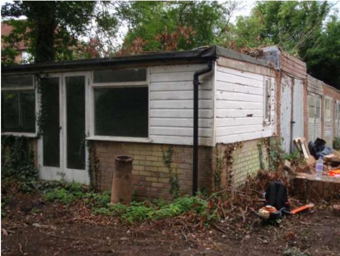
Figure 3. View of site (looking SW)
