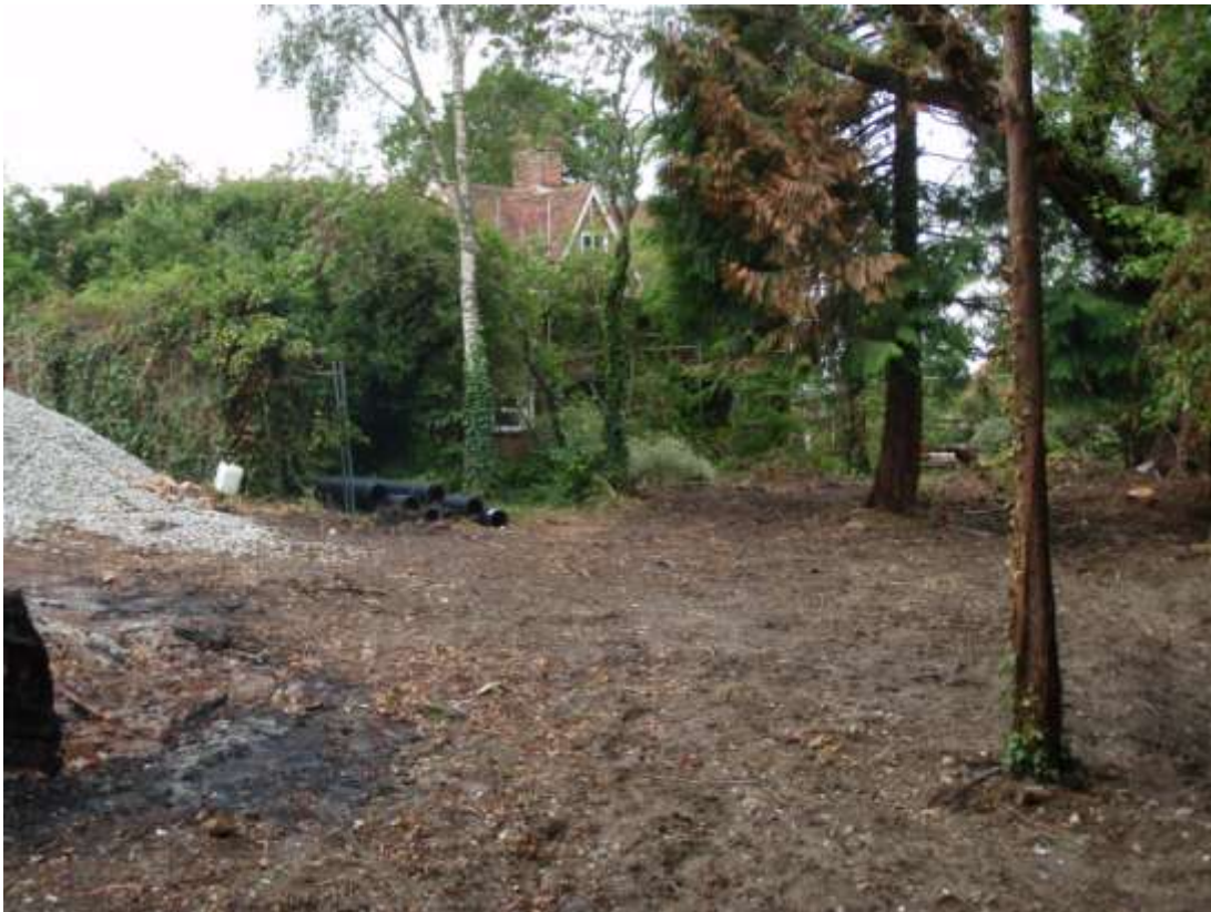
Figure 2. View of site (looking NW)
