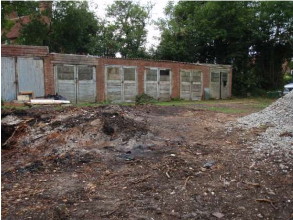
Figure 1. View of site (looking SW)
